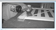
Attach the brace using 2 self-taping screws at each end of the gate as shown here. The screws are provided. Note: Mark the hinge side of socket post with tape. This will keep you from installing the angle brace in the wrong direction.
